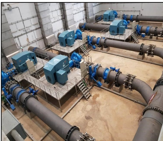
East Water - Pump Replacement
